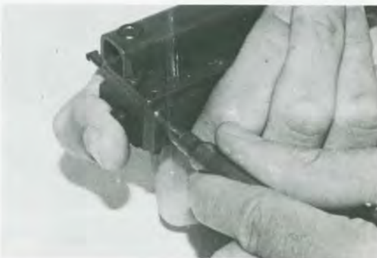
c) Depress firing pin to release cross pin
